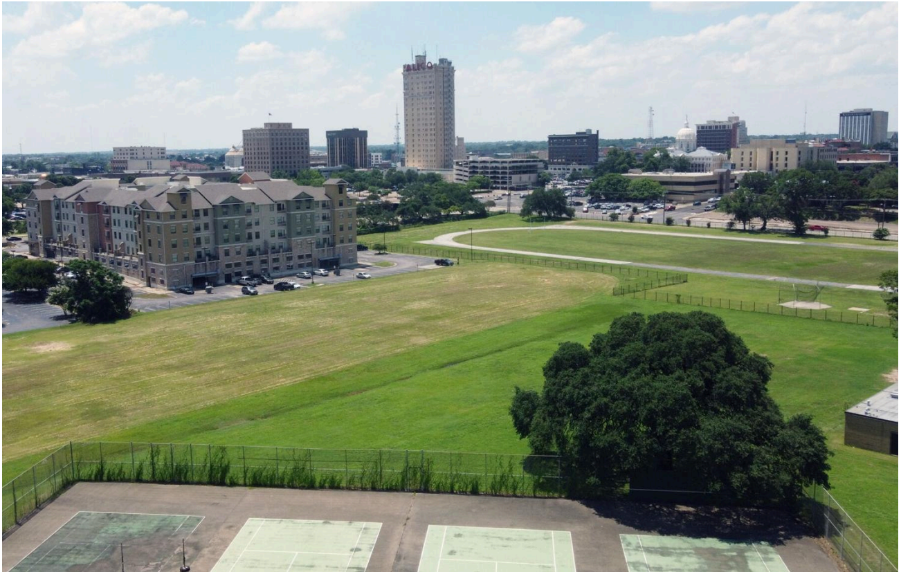
Barron's Branch extends underground through the length of this property, which includes the former Indian Spring Middle School's track. ROD AYDELOTTE, TRIBUNE-HERALD FILE PHOTO
